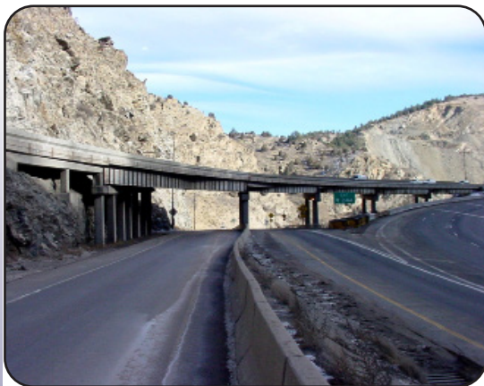
Image 24. I-70 over US6 and Clear Creek in Clear Creek County (F-15-BL)
