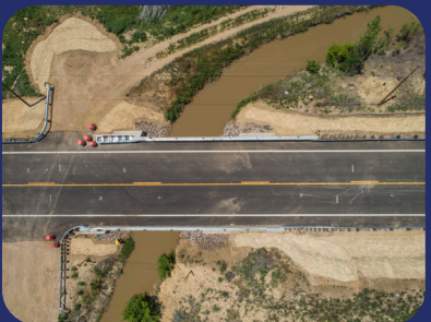
SH 71 ML over Highline Canal in Otero County
