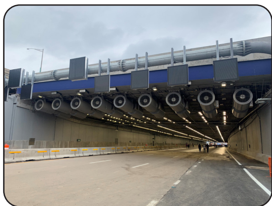
Image 19. Completed Westbound I-70 Lowered Lanes
