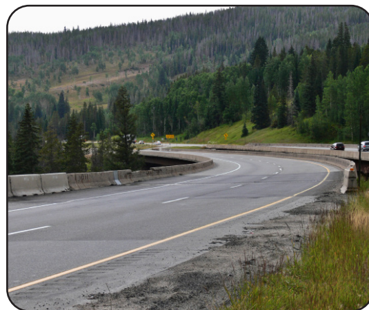
Image 25. I-70 over Polk Creek in Eagle County (F-12-AS)
